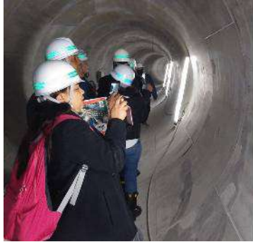
Observation to pump station
