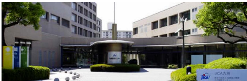
JICA Kyushu Main Entrance
